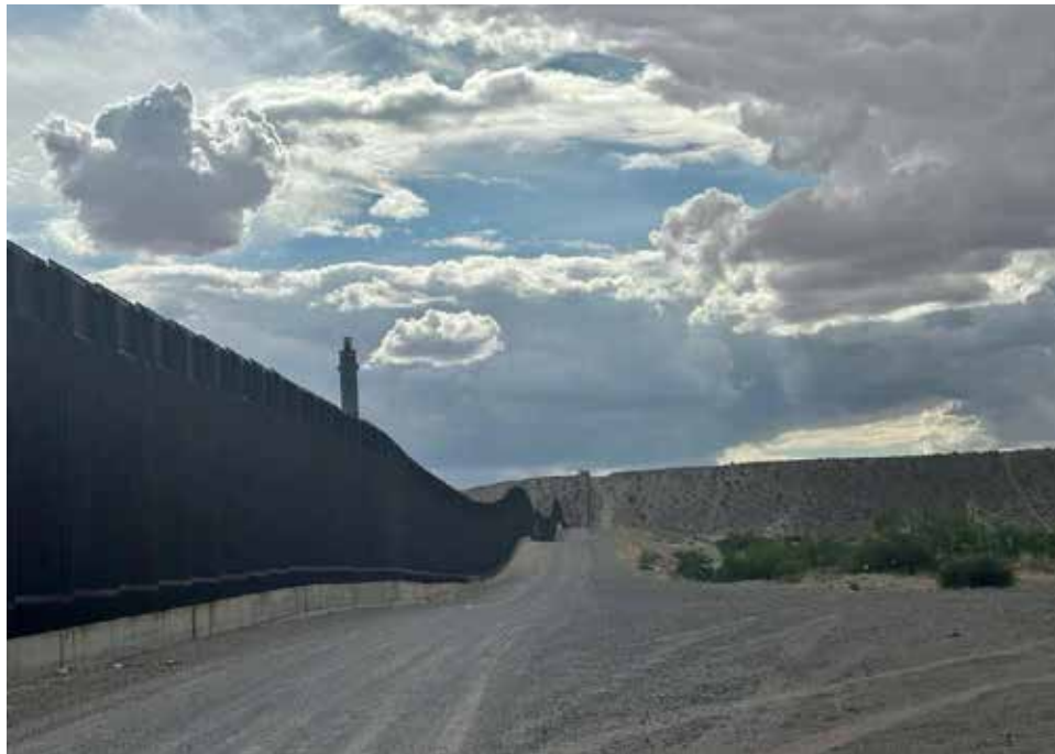
Figure 2. Border Wall South of Texas, April 2023
